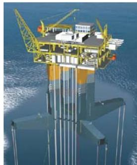
Figura 5 - Plataforma TLP (*Tension Leg Platform*).
